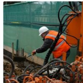
"construction worker in orange safety vest is working on road."
